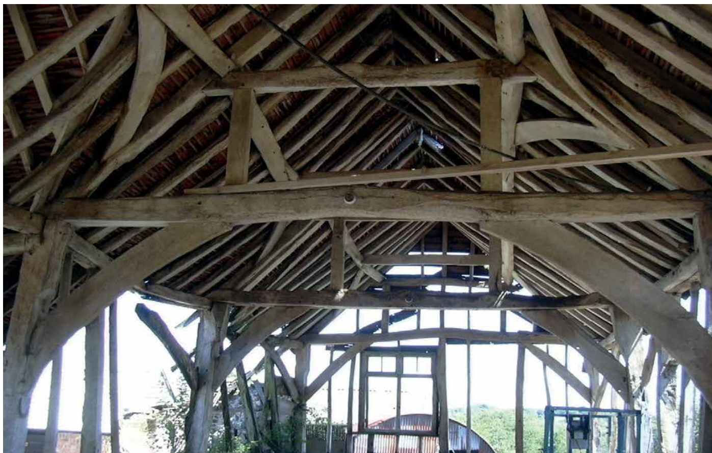
Different types of wood, such as the hardwood pictured, have different properties so it is important to know the species and the source of the wood
