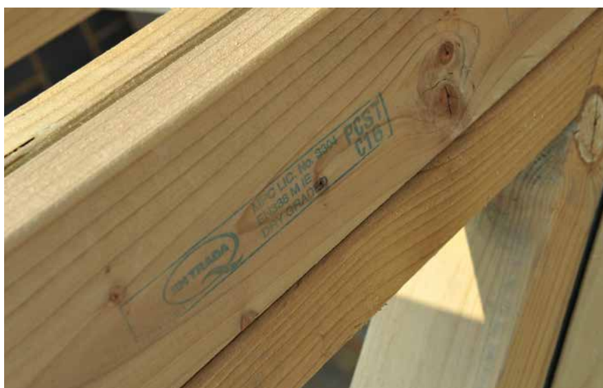
A graded section of timber should display the relevant strength class stamp
