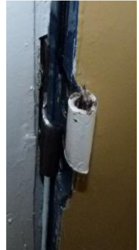
broken butt hinges
