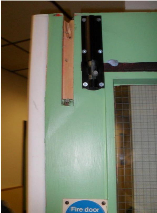
Voids at top of door
