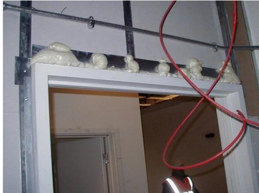
Unprotected foam sealing
